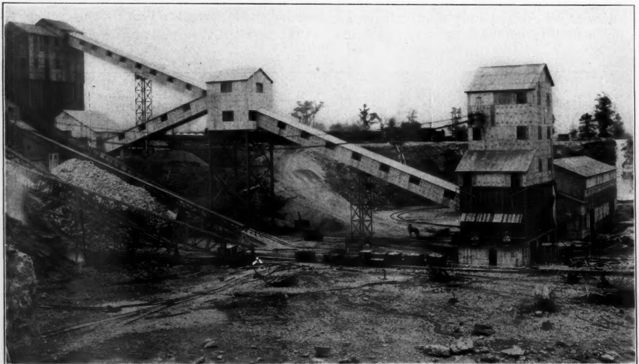
View Showing Crushing Plant in Quarry and Incline.
